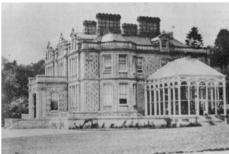
Rosehaugh House c1880. Extensions by Alexander Ross, architect, Inverness
